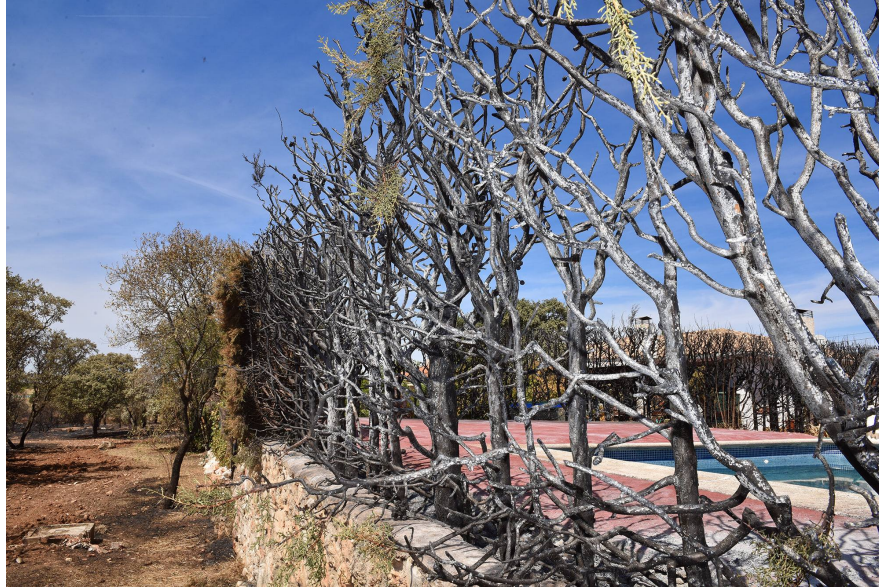
A close view of one of the affected green hedges, receiving the main impact of the left flank. Observe that a separation from the forest fuels was in place, in which the fire reduced intensity. However the flames managed to initiate the combustion and propagation over the garden vegetation.
