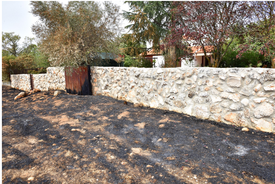
The wall encircling the lot, about 1 m tall, was very effective receiving the flame impact of the surface-propagating fire over the cured grass. This is a very effective design in which the exterior (wall) and the interior of the garden work together to stop the fire and minimize consequences. This should be an example to follow in the rest of the lots in contact with the wildland. It is very clear that lots in the perimeter loaded with flammable vegetation and other materials and objects represent a threat to the rest of the community, as in these points the fire increases intensity and initiates the projection of flying embers. The presence of flammable hedges and undeveloped lots with cured grass in the interior of the community,
