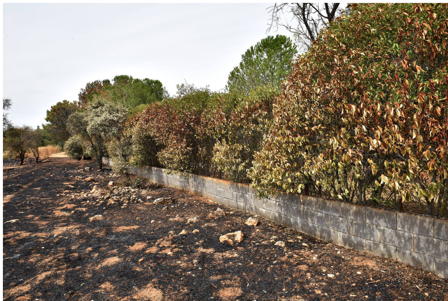
Observe how the presence of a small wall (70 cm) and fire-resistant plants in the lot hedge contributed to reduce the likelihood of the fire jumping inside the parcel and spreading the propagation into the settlement. This is a good example of a proper fire-adapted design of gardens.
