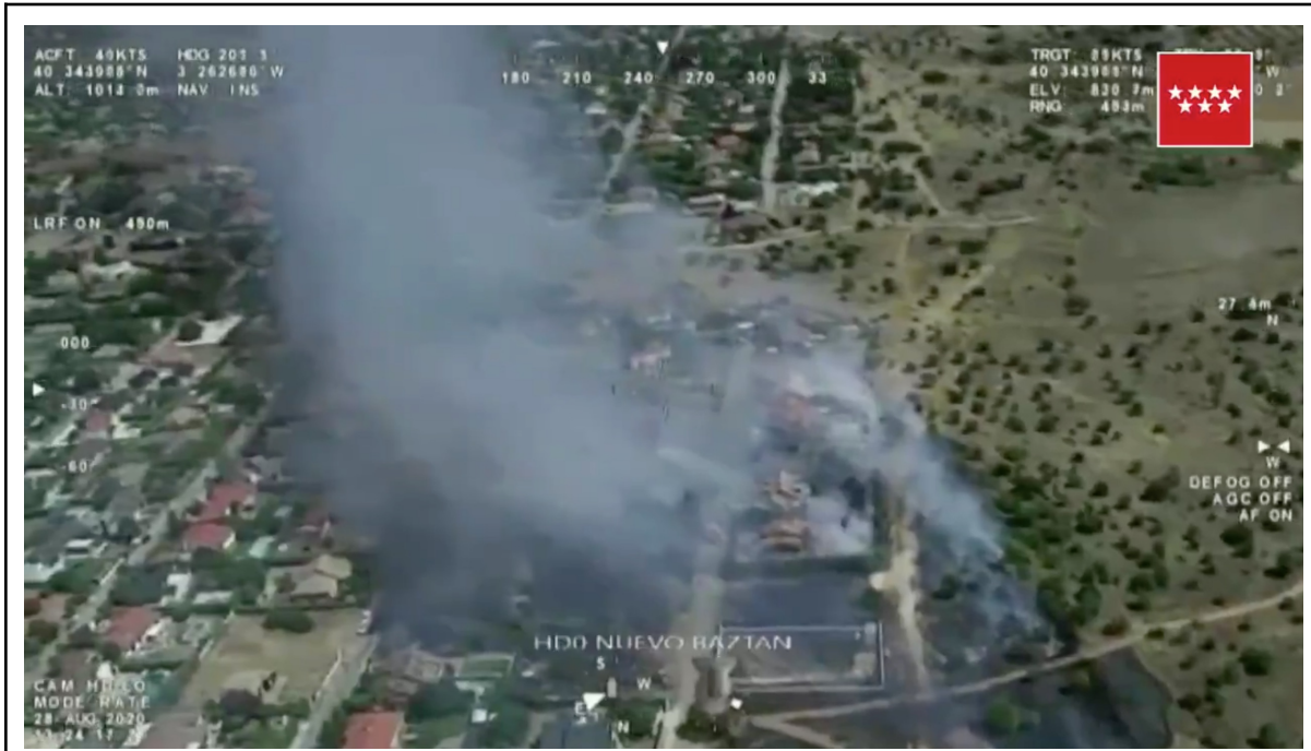
An aerial view of the propagation inside the first and second rows of houses in the settlement, by the time the first aerial means arrived in the area. Note the intensity developed by the gardening elements, more particularly flammable green hedges, and some objects and materials involved, including some vehicles.
