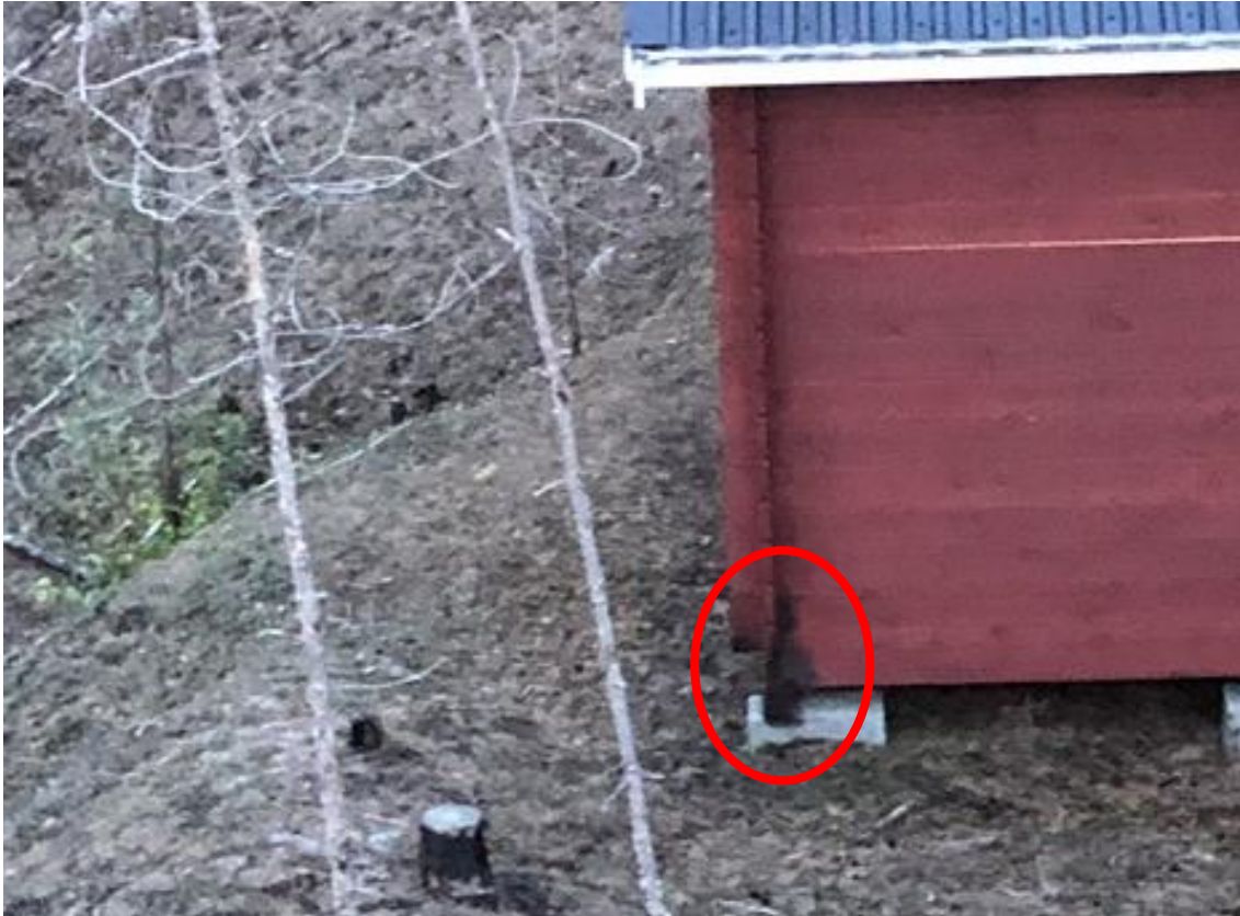
Figure 11. Example of low-intensity fire ignition by flame impingement of the façade, in this case followed by extinction. The vegetation around the structure (below the cover of pine needles) is fully consumed.
